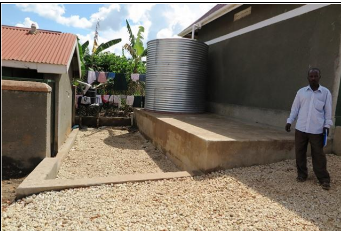
Toilet, rainwater harvesting tank and small stones between the Girls Dormitory and toilet to reach without muddy shoes
